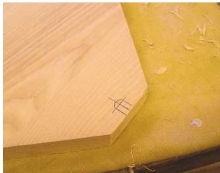
▲ Pic.19 Mark the position of the shelf stud recess by placing each shelf in the cabinet and drawing round it
